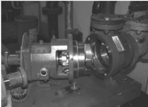
FIGURE 12 BACK PULL-OUT REMOVAL
