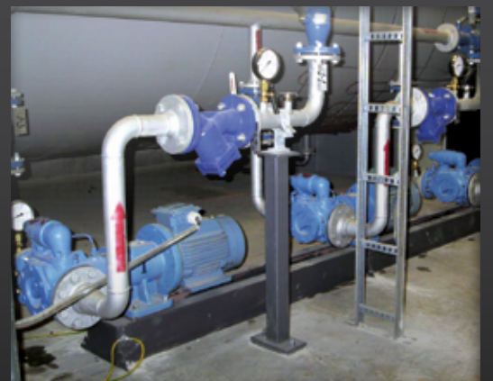
Metric motor speed pumps moving thin liquids in parallel.
