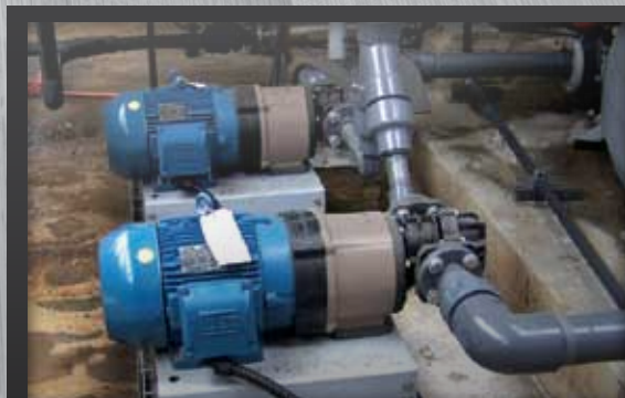
CMD pumps moving chemicals in a series.
